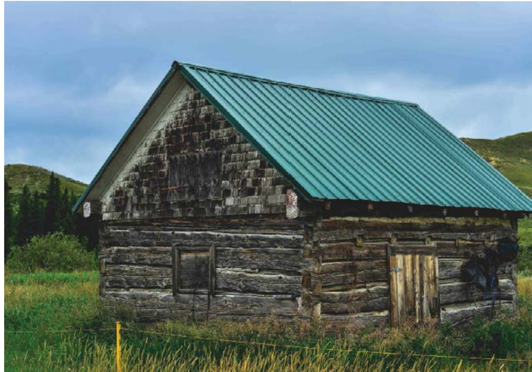
Figure 1.11 Hand Hewn Métis Barn Near Cypress Hills, Saskatchewan, Jason Surkan
